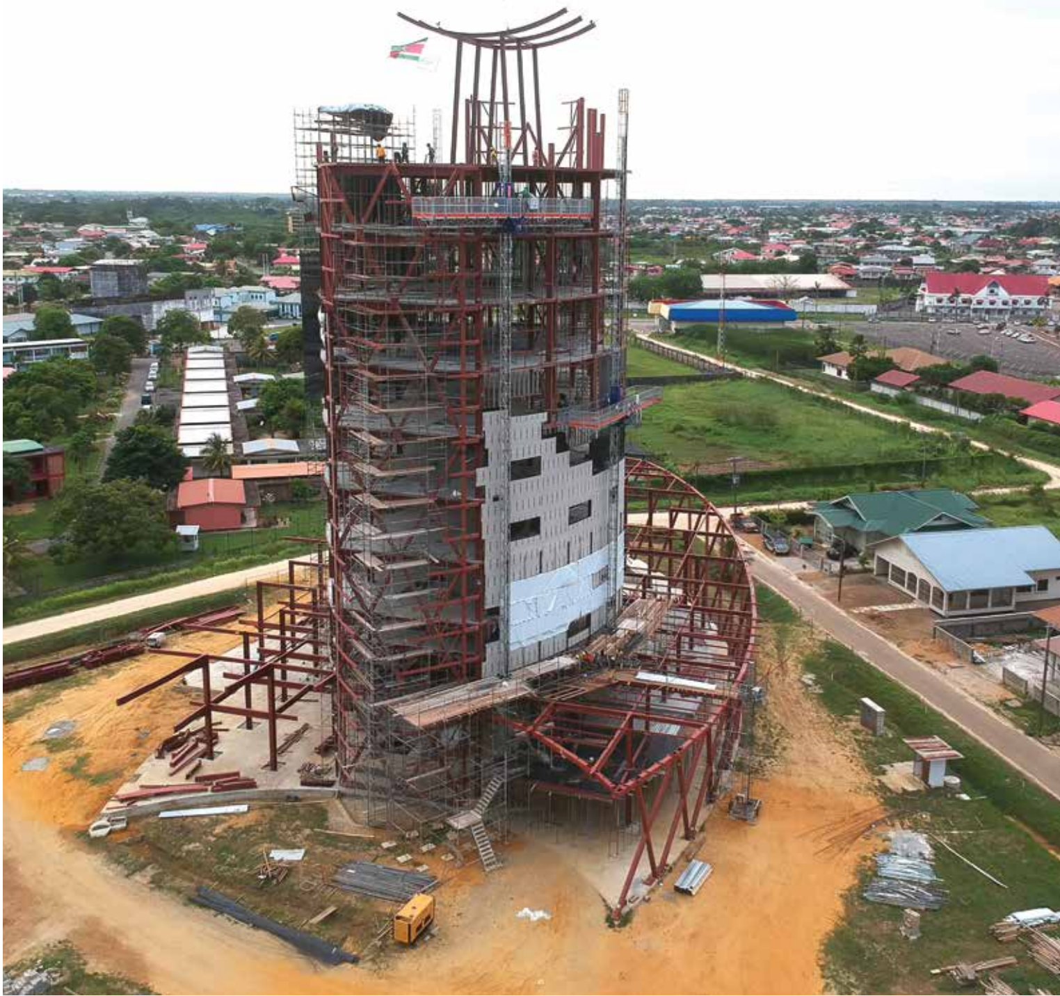
Going up: the Surinamese flag was raised to mark the highest point in construction
