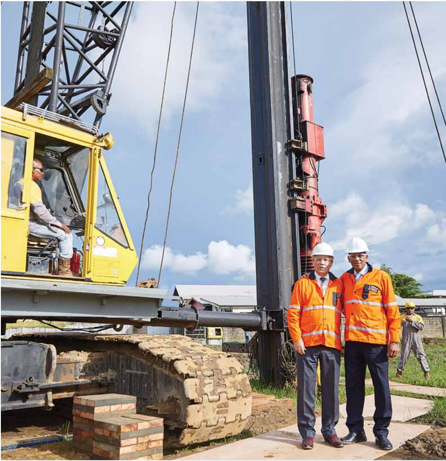
The first milestone of the Assuria Hermitage High-Rise: driving the first pile, one of 265 piles, each one measuring 23 meters long
