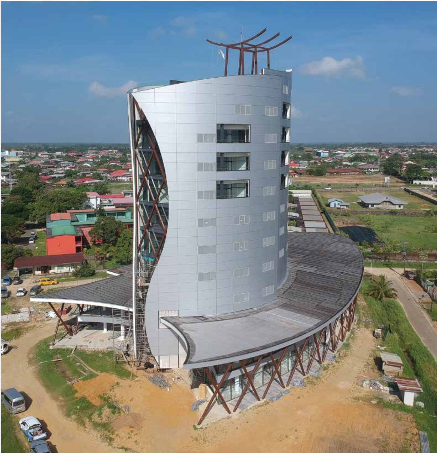
The iconic facade of the Assuria Hermitage High-Rise takes shape when the external wall panels are installed
